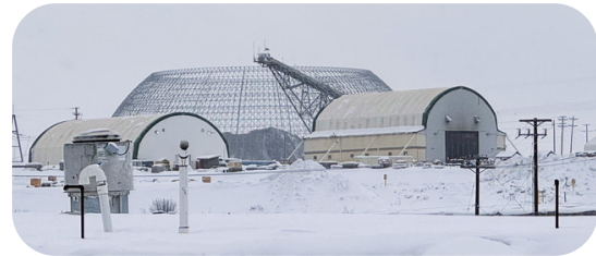
A cover is being installed over the coarse ore stockpile at Red Chris to reduce dust emissions.
