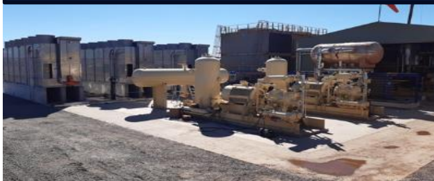
REFRIGERATION PLANT & BULK AIR COOLER
