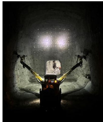
PC1-2 Southern Crusher Chamber Development
