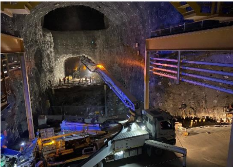
PC2-3 crusher chamber construction
